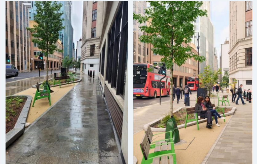
Bevis Marks 'rain garden' a SUDs project planted in an engineered substrate.
